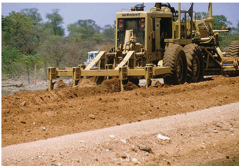
Figure 17-18: Use of grader tines for effective mixing of water in material
