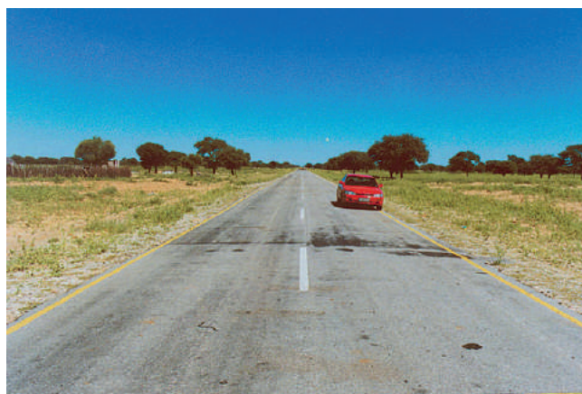
Figure 17-12: Example of poor transverse joint construction
