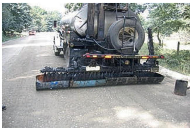
Figure 17-11: Example of poor transverse distribution of binder
