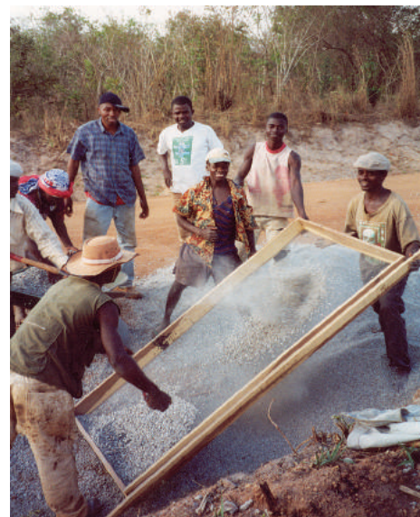
Figure 17-2: Screening of aggregate for road surfacing using labour
