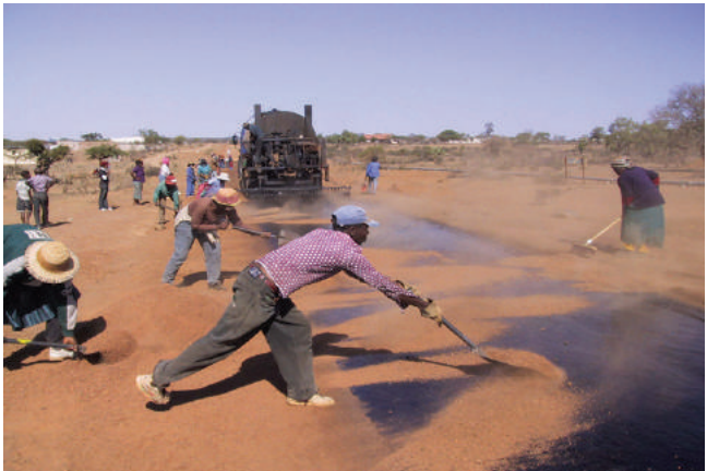
Figure 17-16: Spreading gravel using labour-based methods for an Otta seal
