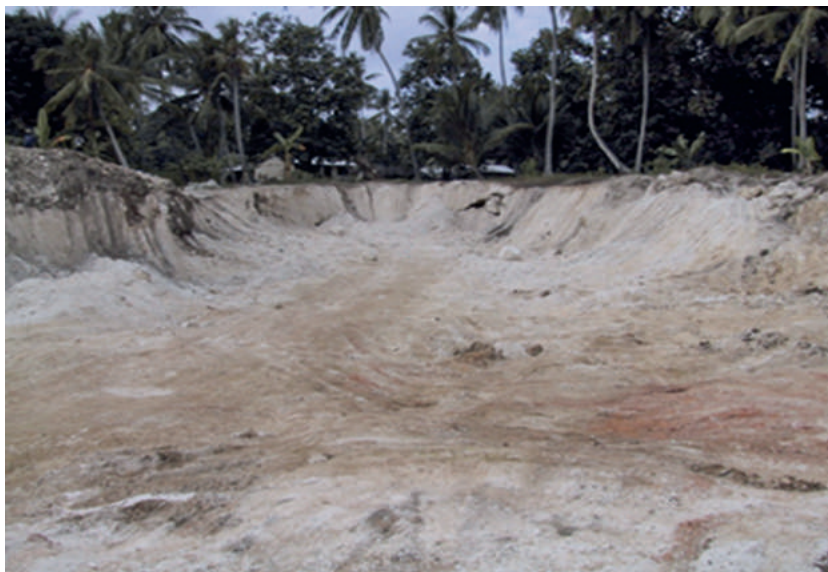
Figure 18-1: Near surface natural gravel borrow pit containing calcrete (Pemba island)
