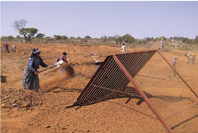
Figure 17-15: Screening of aggregate using labour-based methods
