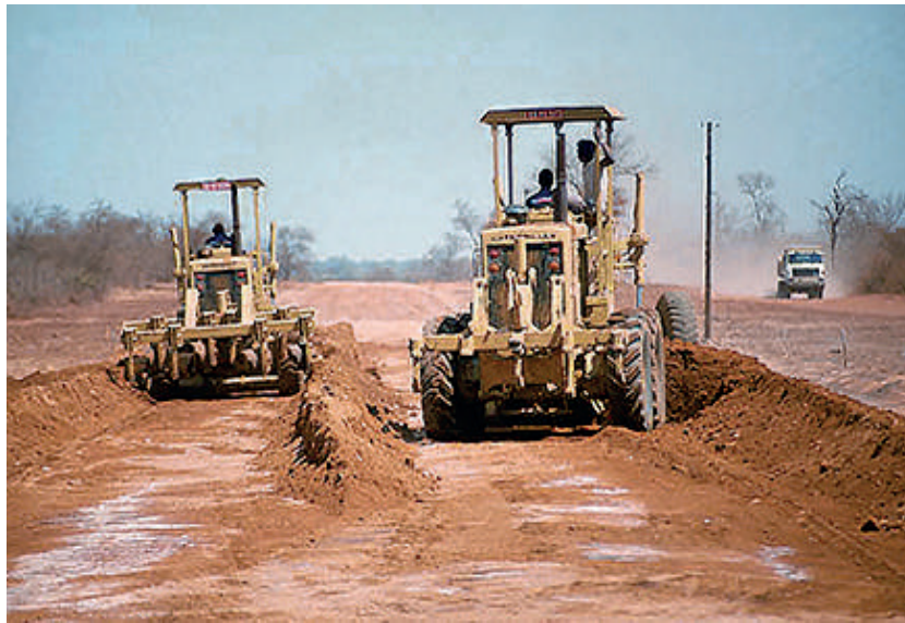
Figure 17-7: Material processing using motor graders
