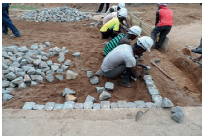
Figure 17-13: Construction of cobble stone paving
