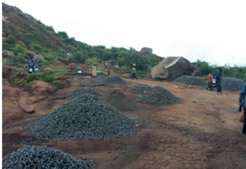
Figure 18-5: Aggregate crushed by LBM
