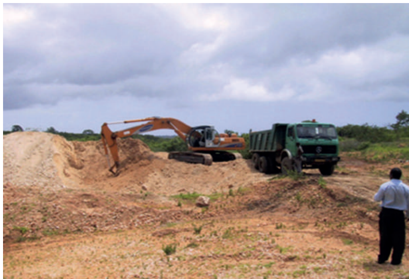
Figure 18-6: Shallow borrow pit excavation using machine based methods
