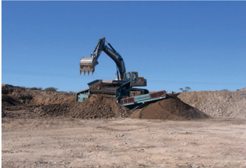
Figure 18-17: Mobile vibrating screen used to remove oversize aggregate in the borrow pit
