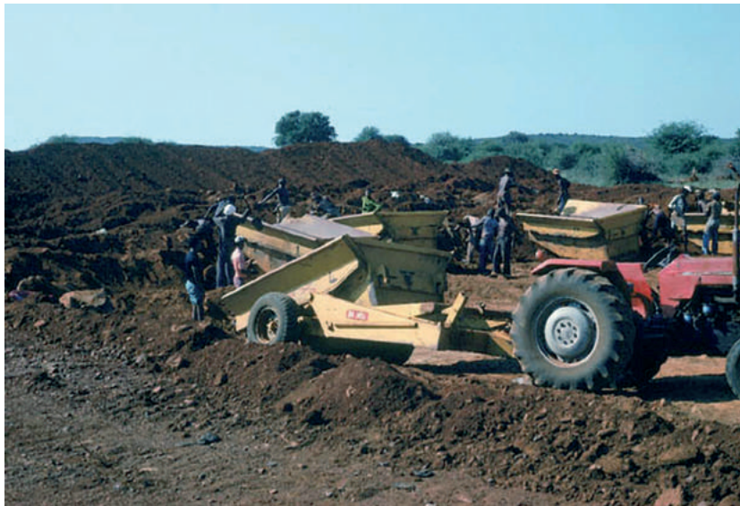
Figure 17-6: The use of small tractor-drawn trailers in labour-based construction
