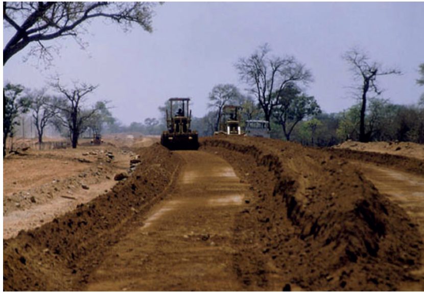
Figure 17-10: Mixing material on road with a motor grader
