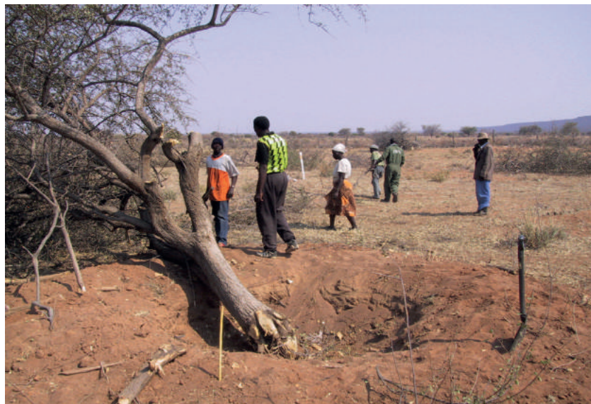
Figure 17-1: De-stumping of trees using labour-based methods
