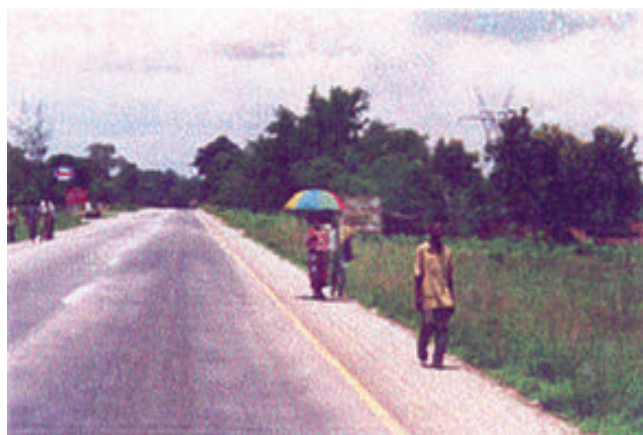
Figure 10-9: Sealed shoulder used to cater for pedestrian or NMT
