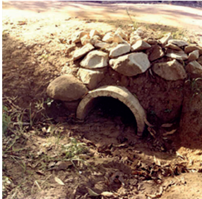
Figure 11-8: Siltation problems
