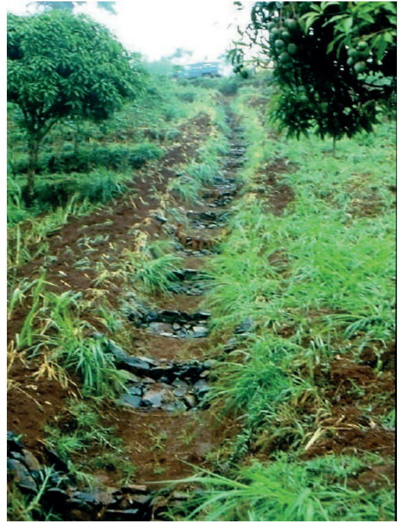
Figure 12-20: Grassed waterway with check dam
