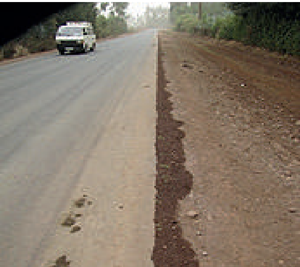
Figure 12-4: Infiltration of water through a permeable surfacing
