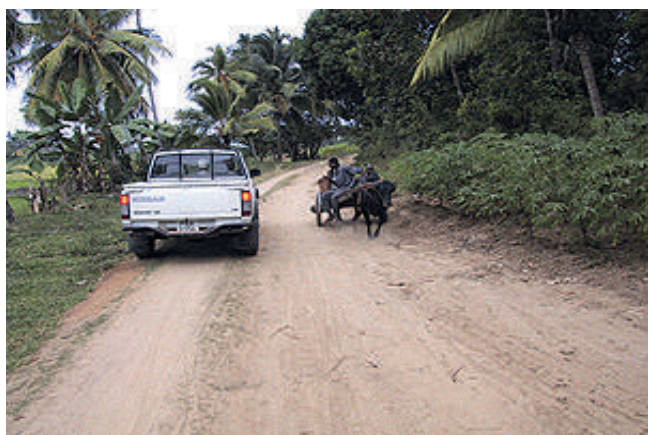
Figure 10-4: Problems encountered on unpaved road
