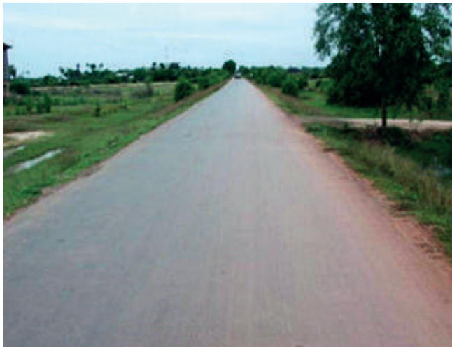
Figure 16-7: Paved road option (Higher construction costs, lower maintenance and road user costs)
