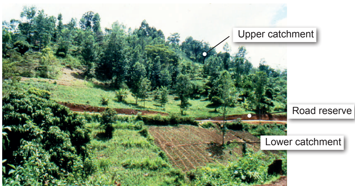
Figure 12-14: Erosion areas—upper catchment, road reserve and lower catchment
