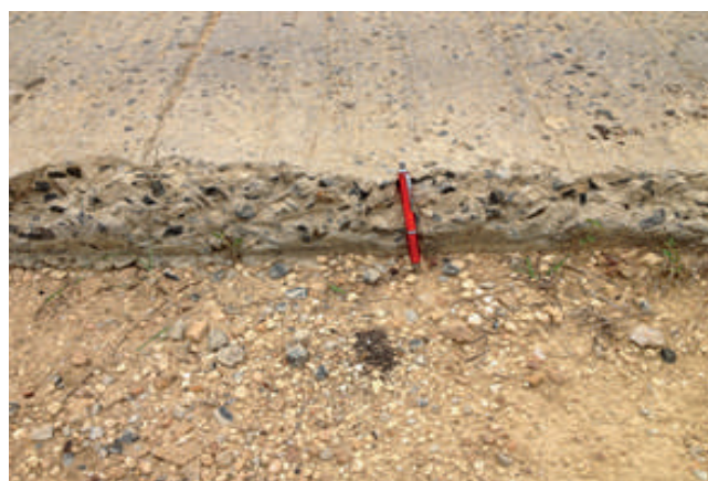
Figure 15-9: Concrete strip road with dangerous edge drop
