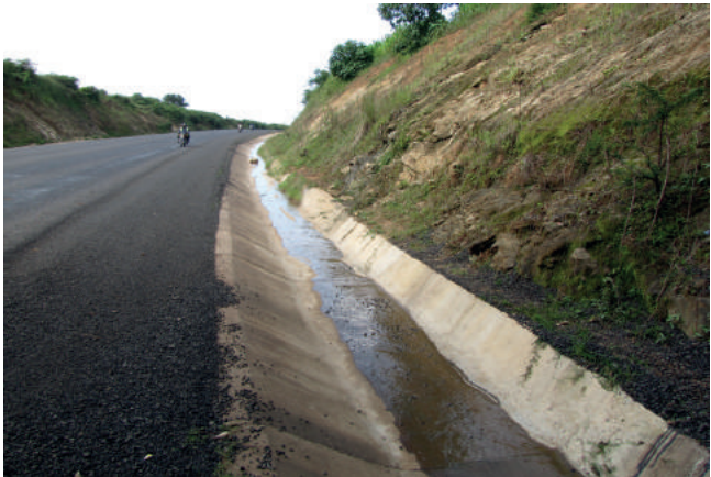
Figure 12-18: Concrete lined drain
