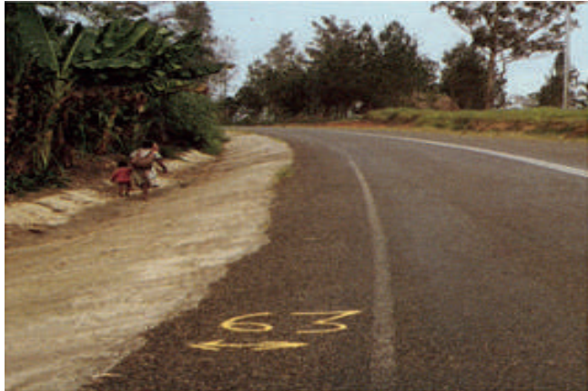
Figure 10-12: Well designed roadside drain (Shallow side slopes improve safety)
