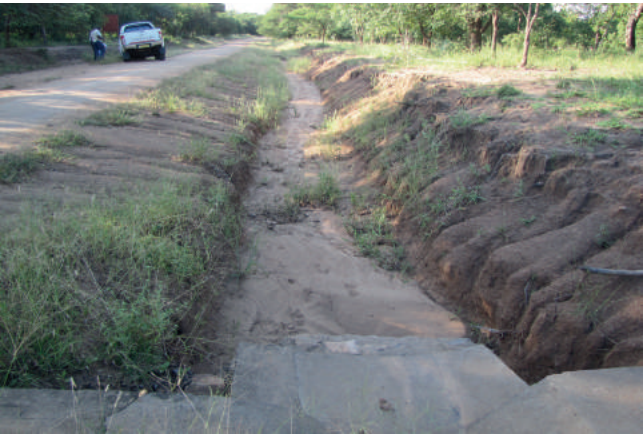
Figure 12-17: Severe erosion
