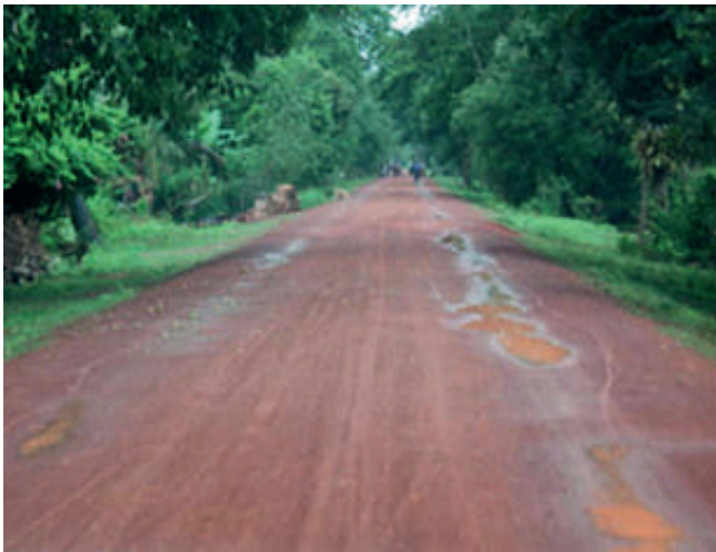
Figure.16-6: Gravel road option (Lower construction costs, higher maintenance and road user costs)
