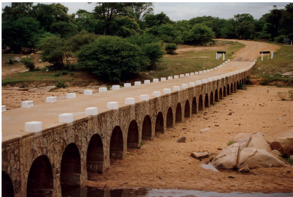
Figure 11-10: A typical vented drift / causeway
