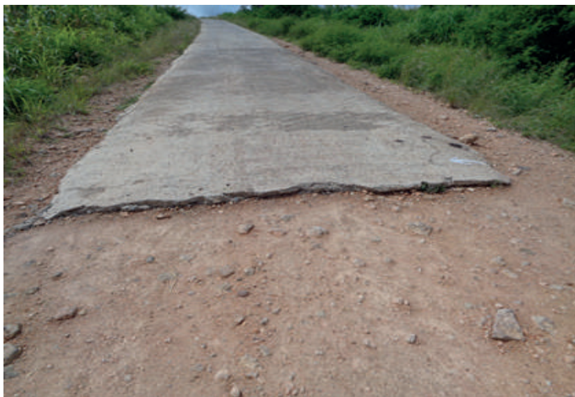
Figure 15-10: Example of two different adjoining surfacings with dangerous edge drop
