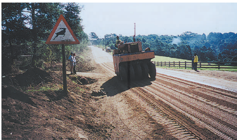
Figure 15-5: Extensive rolling of an Otta Seal- essential to achieve a good result
