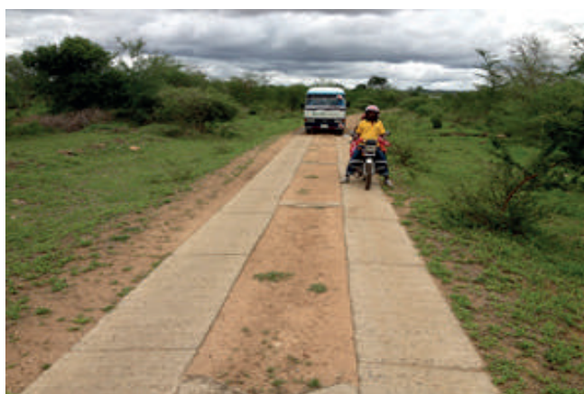
Figure 15-9: Concrete strip road with dangerous edge drop
