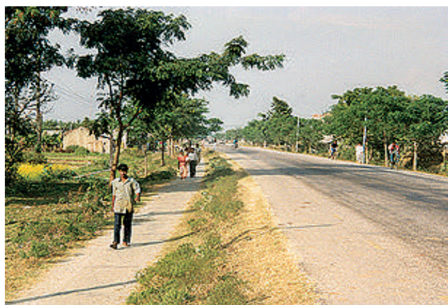
Figure 10-7: Segregated footpath off road (Cost effective means of catering for high volumes of pedestrian traffic)
