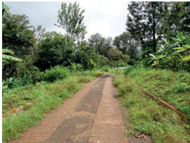
Figure 10-19: Example of poorly maintained concrete strip road
