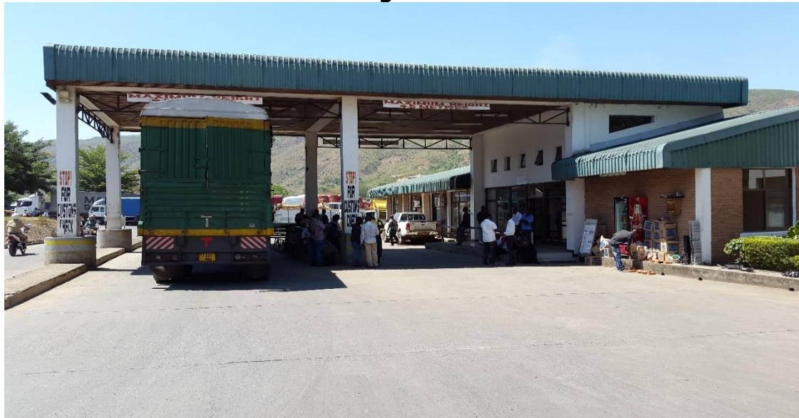
Picture 1: Kasumulu Transit charges collection Point
