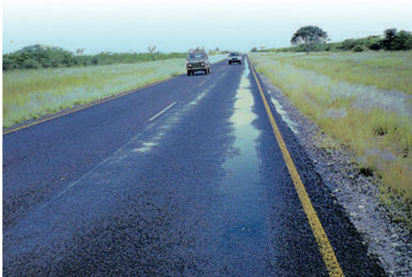
Figure 6-11: Typical manifestation of collapsible subgrade
