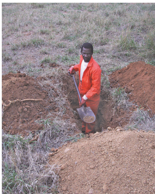
Figure 5-3: Test pits for LVRs are commonly excavated using labour
