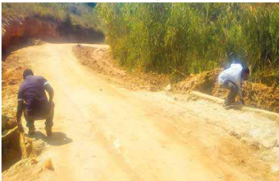
Picture 1 1: Technical Auditor verifying road width during Preventive Technical Audit
